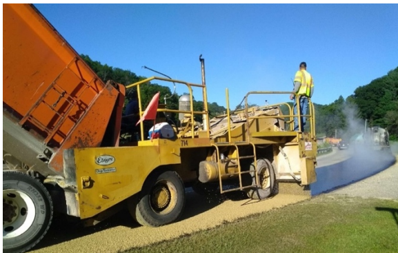
Wheel tax revenues are being used to seal coat County highways, like County Highway D near West Lima.
