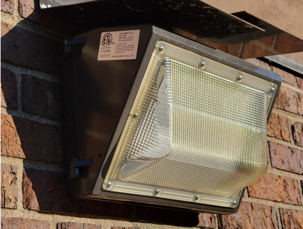
FIGURE 4 HOCAN WAL PAK FIXTURE ON SCIENCE BUILDING AT CAMPUS SITE
