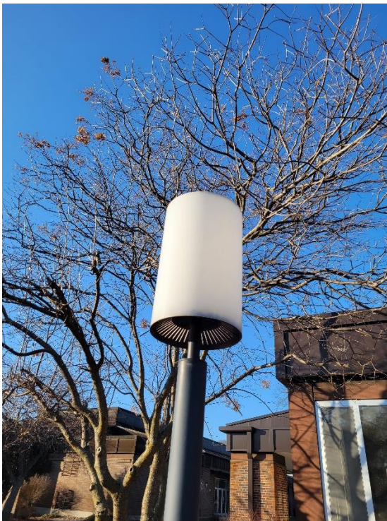
FIGURE 2 WALKWAY LIGHTING AT CAMPUS SITE
